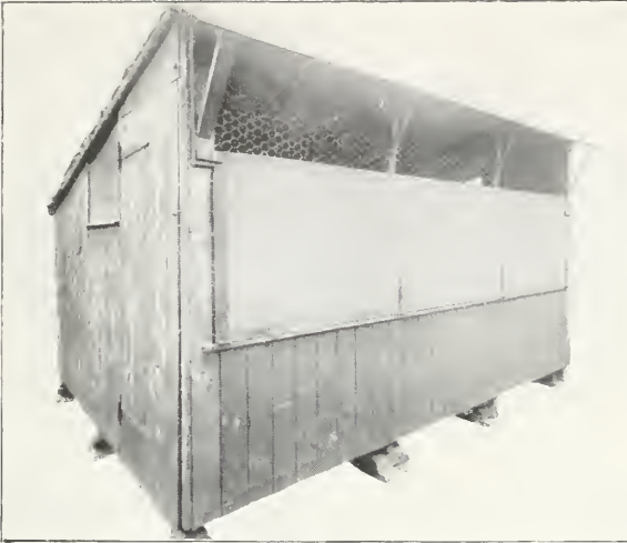
House for 30 Birds on Mrs. Baynes's Intensive Plant showing Rain-shutter Up. Note the Overhanging Drip-board at Top.
